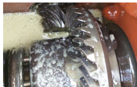
Surface foam in a gear unit
